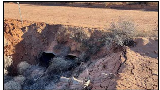
Culvert Cross Drain
