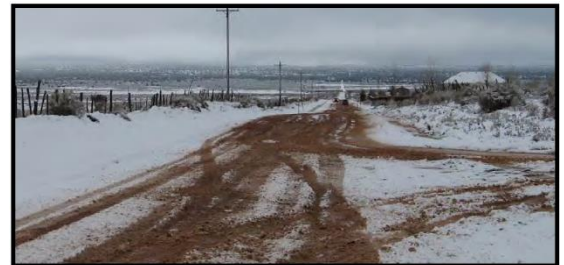
Cane Beds Road Post-Storm Condition
